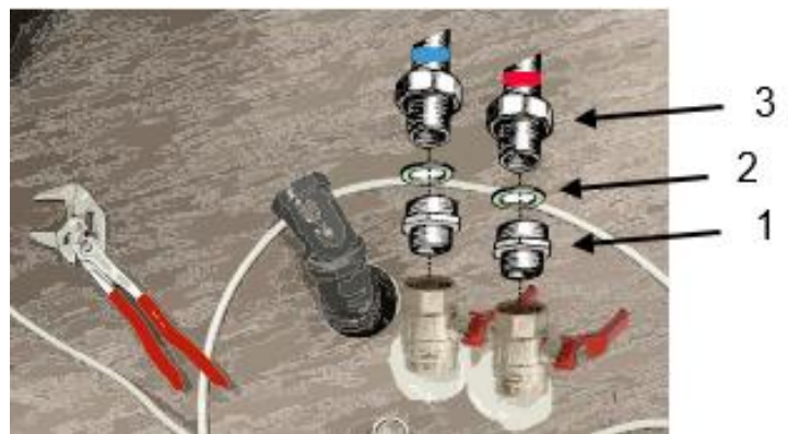
Figure 2 Connection water pipes.
